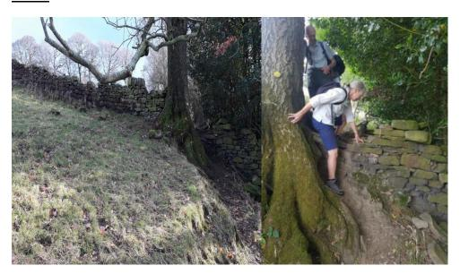
Description of existing structure – Collapsing drystone wall and low hanging tree bough
