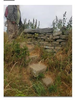
Description of existing structure - Steep, worn, sloping steps
