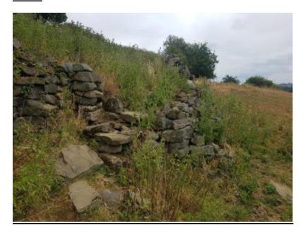
Description of existing structure - Collapsed stone stile and length of wall
